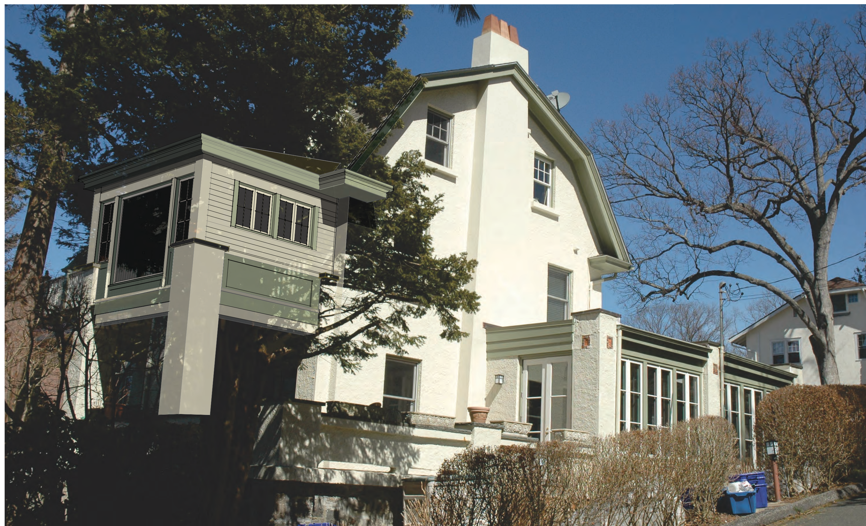
2 SOUTHWEST ELEVATION VIEW
