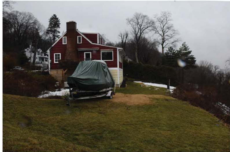
3. NORTH WEST - VIEW FRPOM PRIVATE LAND
