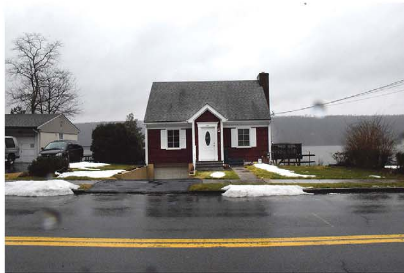
4. STRAIGHT ON VIEW FROM WARBURTON AVE
