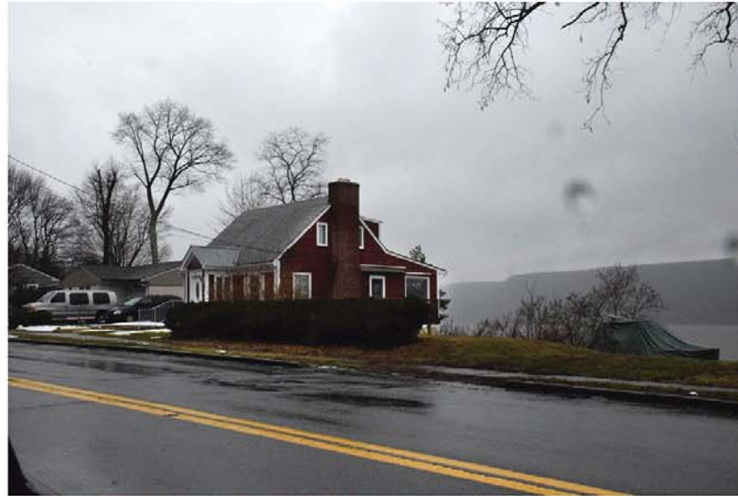
2. NORTH EAST VIEW FROM WARBURTON AVE
