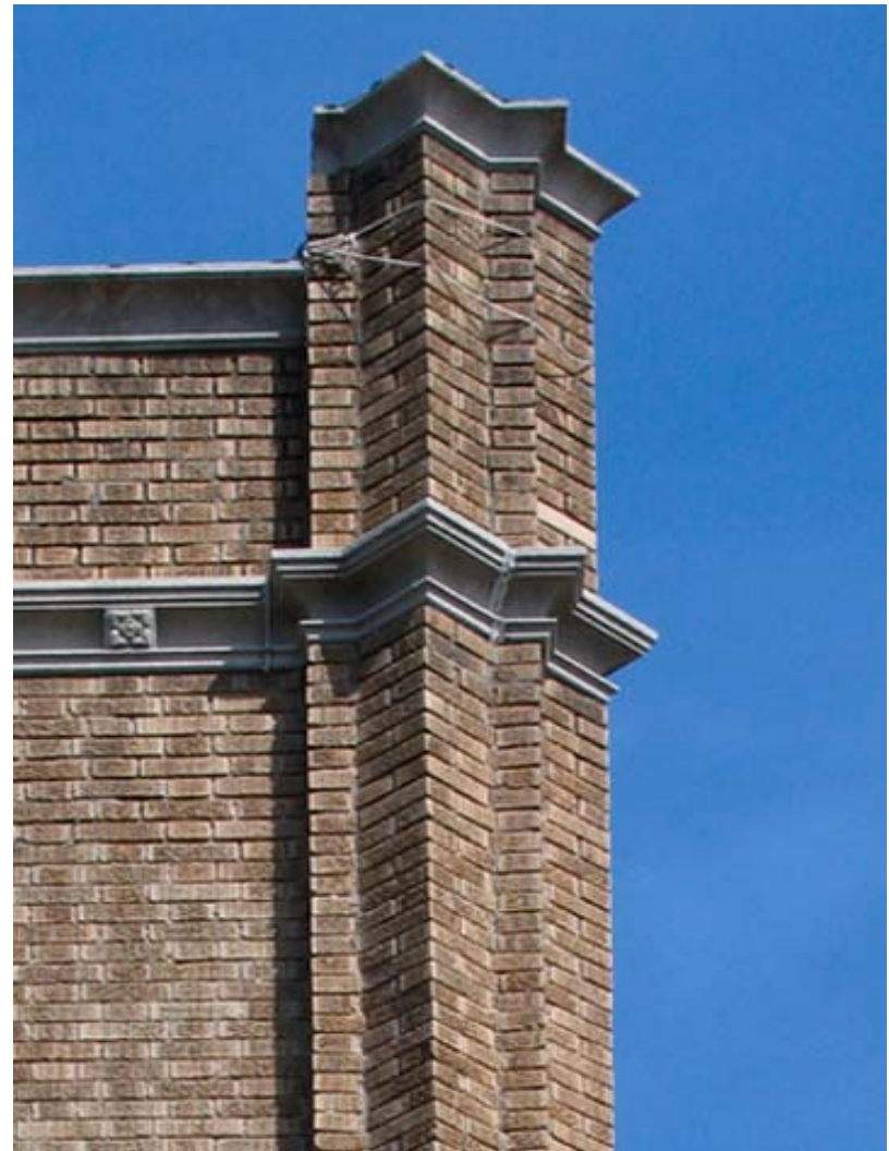
Parapet Detail on Warburton Avenue
