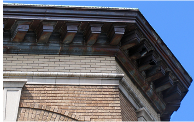
Cornice Detail at 555 Warburton Avenue
