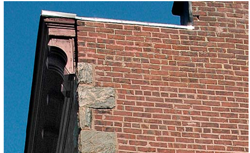
Parapet Detail on Main Street
