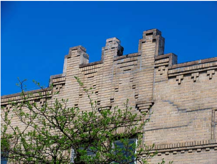
Parapet Detail on Warburton Avenue
