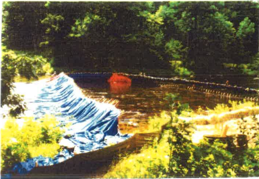
The Tennessee Gas Pipeline Company installed a cofferdam across the Farmington River to allow digging to replace its pipeline.
