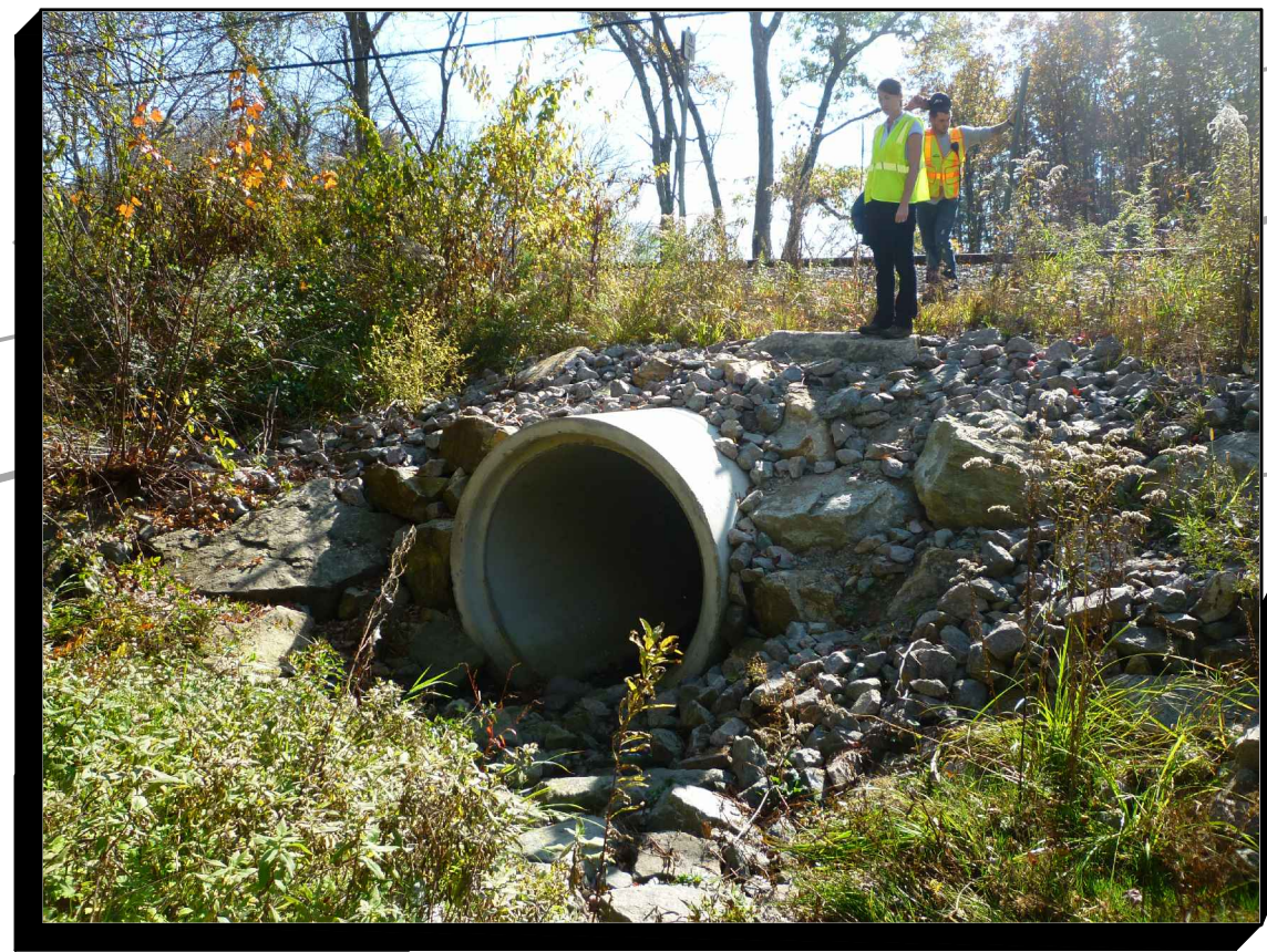
EXISTING 60" DIA CULVERT UNDER RAILROAD (DOWNSTREAM SIDE)
