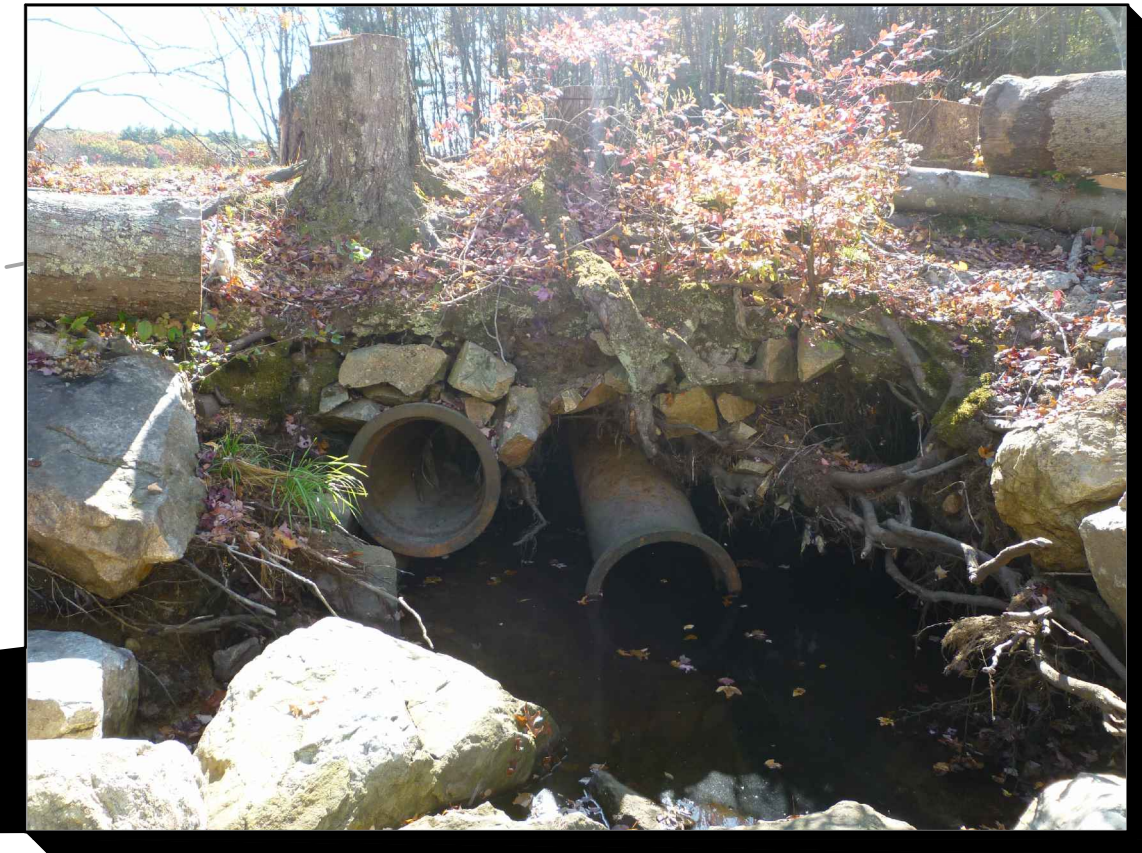
EXISTING 20" DIA. CULVERTS UNDER BEAVER STREET INTERCEPTOR (UPSTREAM SIDE)
