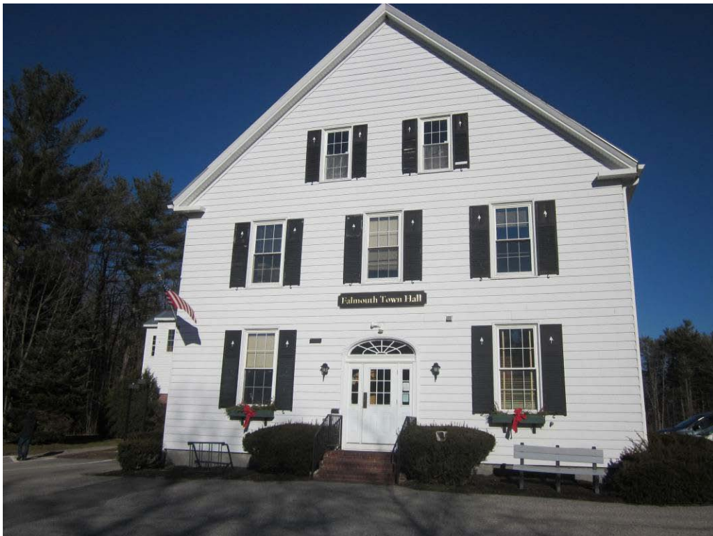
Photo 10 - Town Hall - current asbestos siding
