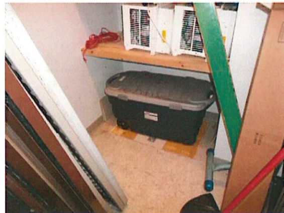
Access to the crawlspace in Council Chambers closet
