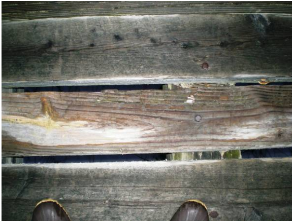
Photo 7 – Green mildew growing on top surface of stringer as seen between gaps in deck boards.
