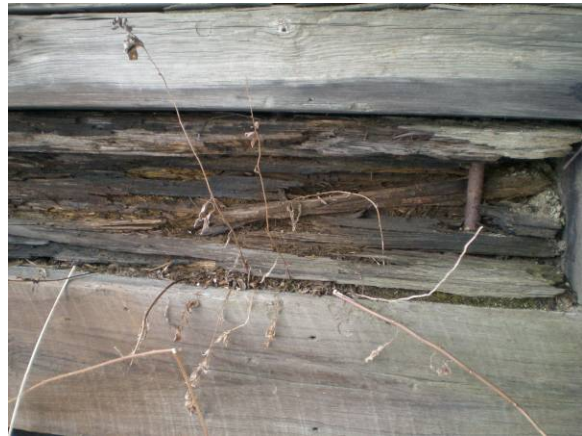
Photo 10 – Deteriorated wood can be removed by hand from abutment timbers.
