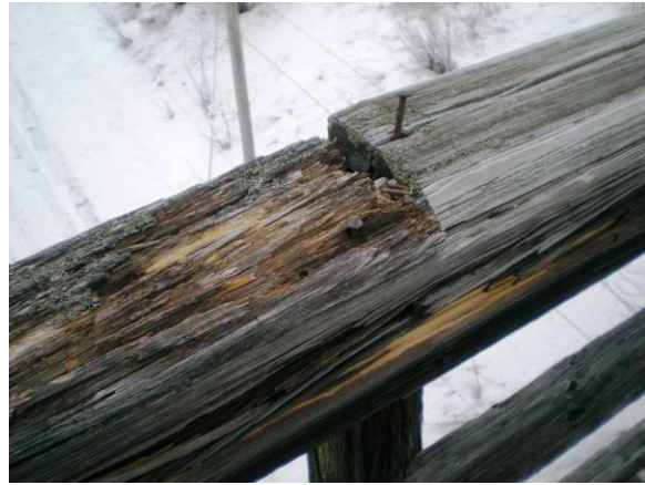
Photo 2 – Top railings are deteriorated and loose at several locations.
