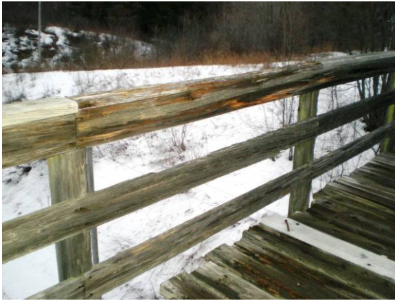
Photo 1 – Deteriorated bridge railing. Spacing of horizontal rails exceeds code required 4" maximum.
