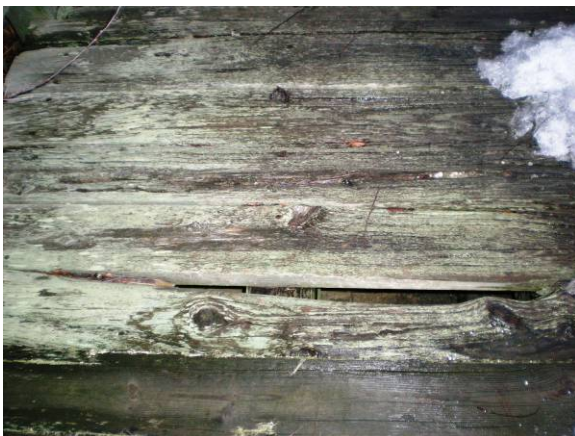
Photo 5 – Moss, mildew, and decay on deck boards.
