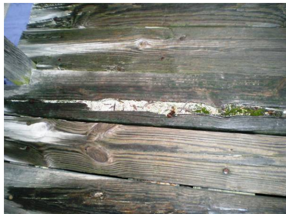
Photo 6 – Cracked deck board with moss growing.
