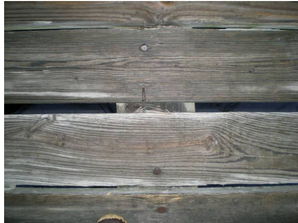
Photo 8 – Moisture tends to collect on top surface of stringers at deck boards.
