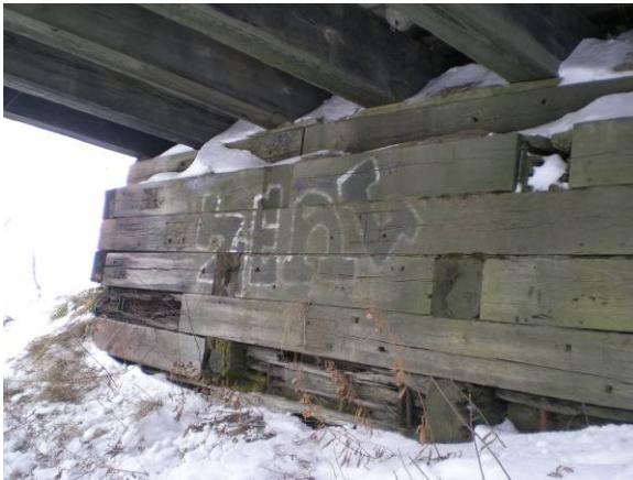
Photo 9 – Severely deteriorated lower timbers of the abutment closest to the shopping center.
