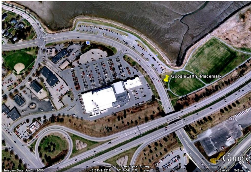
FOREST AVENUE HANNAFORD SHOPPING CENTER WITH WHITE "COOL" ROOF
