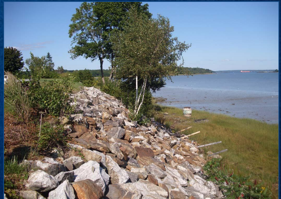
Well-sorted rip-rap stabilization at McKinley.
