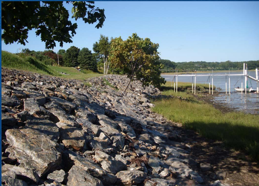
Well-sorted and terraced rip rap stabilization at Hammond.
