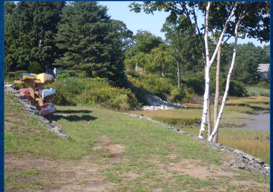
Well-sorted and terraced rip rap stabilization at Hammond.
