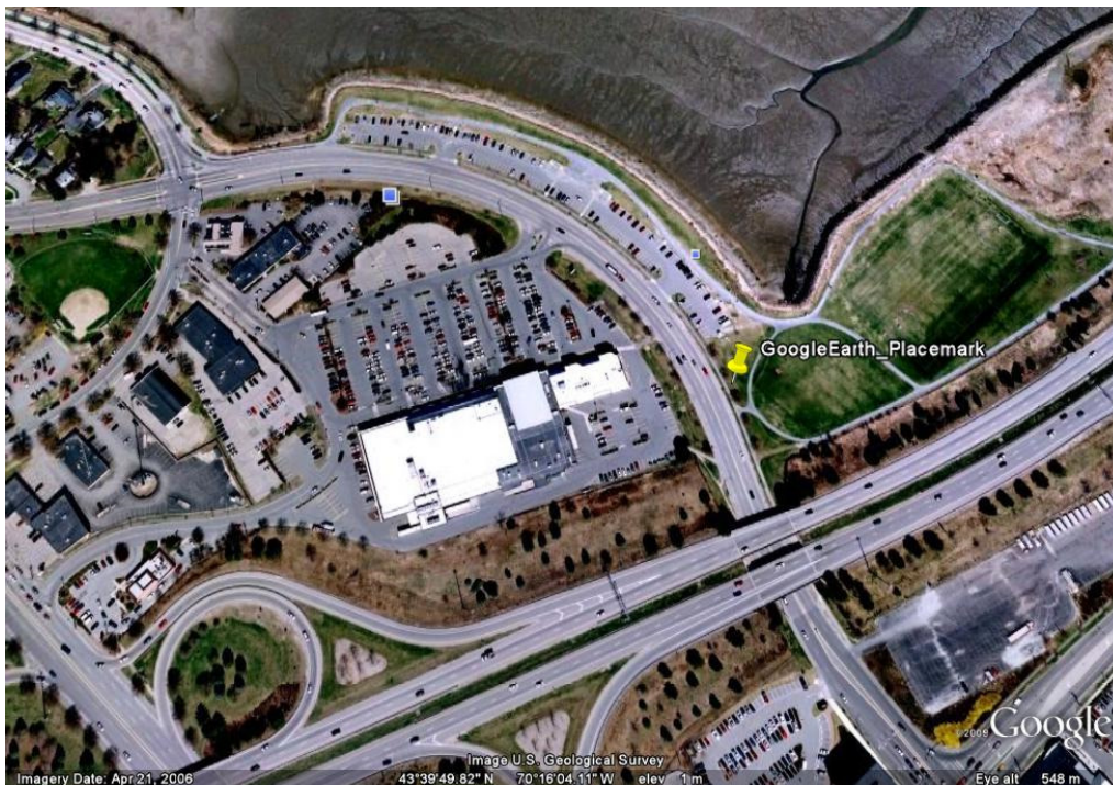
FOREST AVENUE HANNAFORD SHOPPING CENTER WITH WHITE "COOL" ROOF
