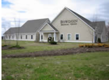
Bowdoin Medical Group building
