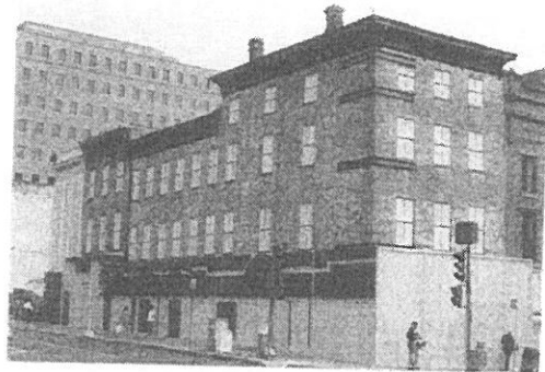
Figure 11. Urban buildings often need additional protection from unwanted entry and graffiti. This commercial building uses painted plywood panels to cover expansive glass storefronts and chain link fencing is applied on top of the panels. The upper windows on the street sides have been covered and painted to resemble 19th century sash. Photo: Thomas Jester, NPS.
