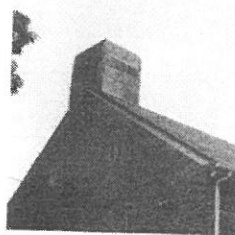
b. Plywood panels stabilize the chimneys. Note the gable vents.
