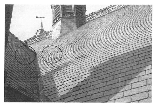
We found several areas of the roof which will require repair. Many of the slate tiles have moved and need refastening; in some cases, the slates are missing. These areas, noted in the two highlighted ovals above could account for the damage currently seen in the auditorium. The valley flashing seen in the picture above was replaced in 2000 and should not be a problem. Many slates
