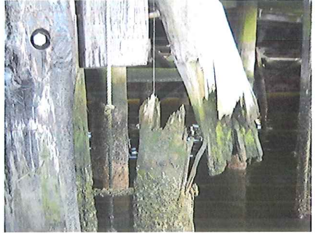
Broken Piling
