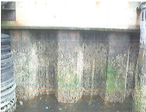
South Side – Steel Bulkhead
