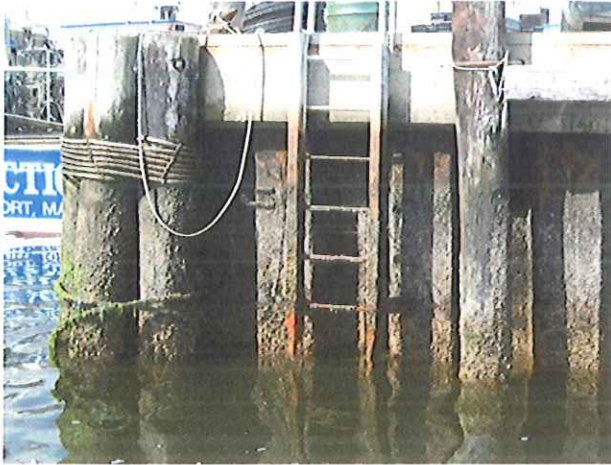
West Side - Steel Bulkhead at South Corner
