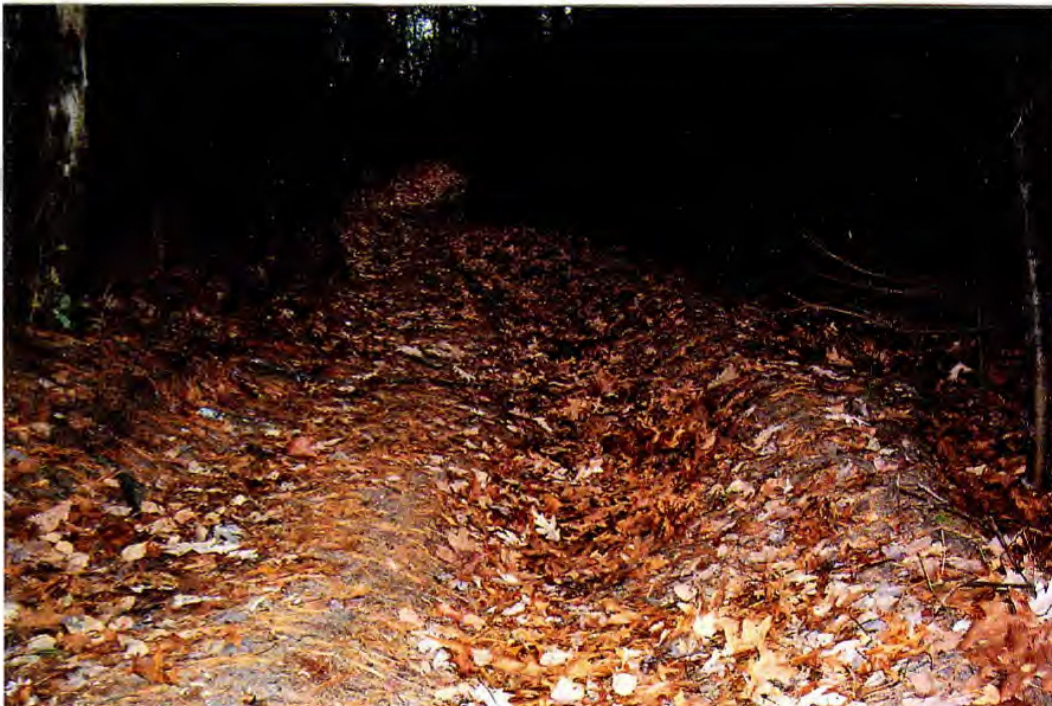
Town Forest: Deep rutting caused by excessive speed on one of the permanent roads.
