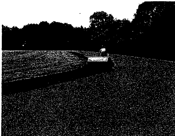
Polyresin Surface Application
