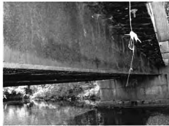
Figure 5: Girder 5 looking East
