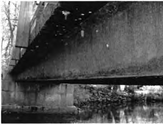
Figure 4: Girder 1 looking East
