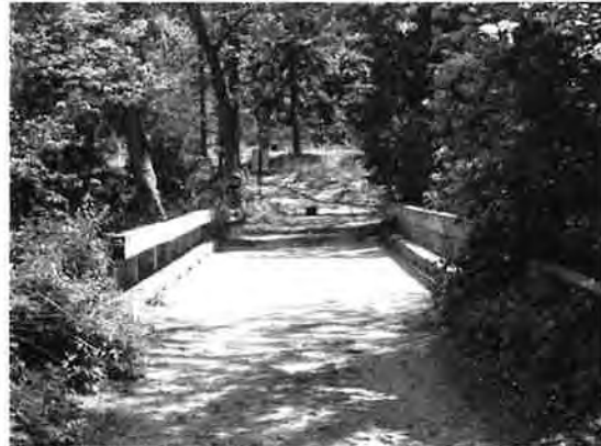
Figure 3: Bridge looking East
