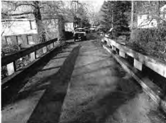
Figure 2: Bridge looking West
