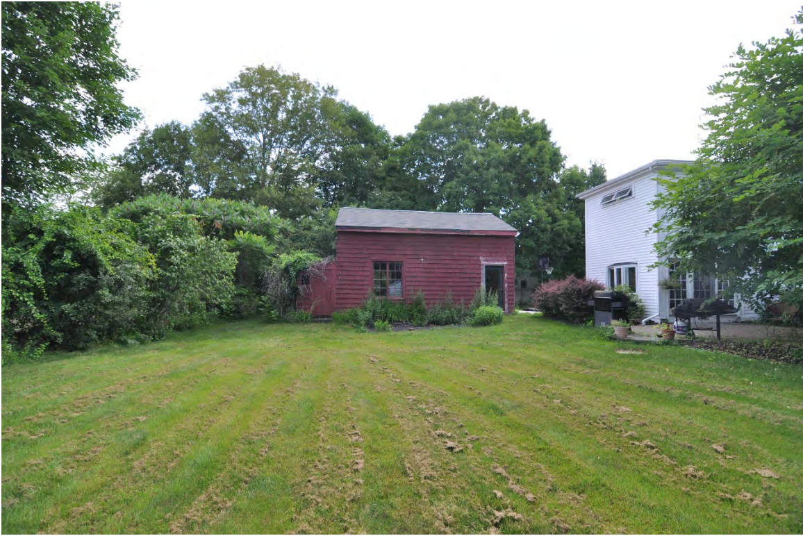
183 Washington Street – view from SIDE (West)
