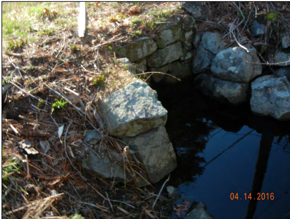
Photo No. 8 – 18” RCP pipe between northwest wetland and Kelsey Road wetland (1,200 feet upstream of Kelsey Rd. culvert under railroad roadbed)
