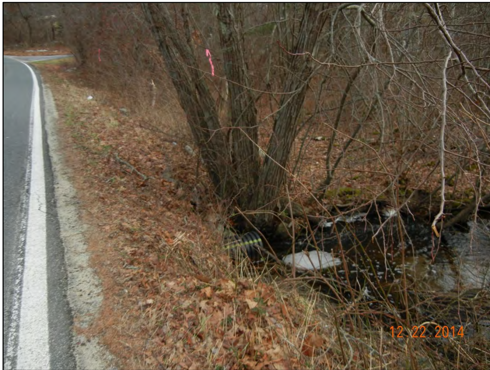
Photo No. 1 – Downstream culvert end
