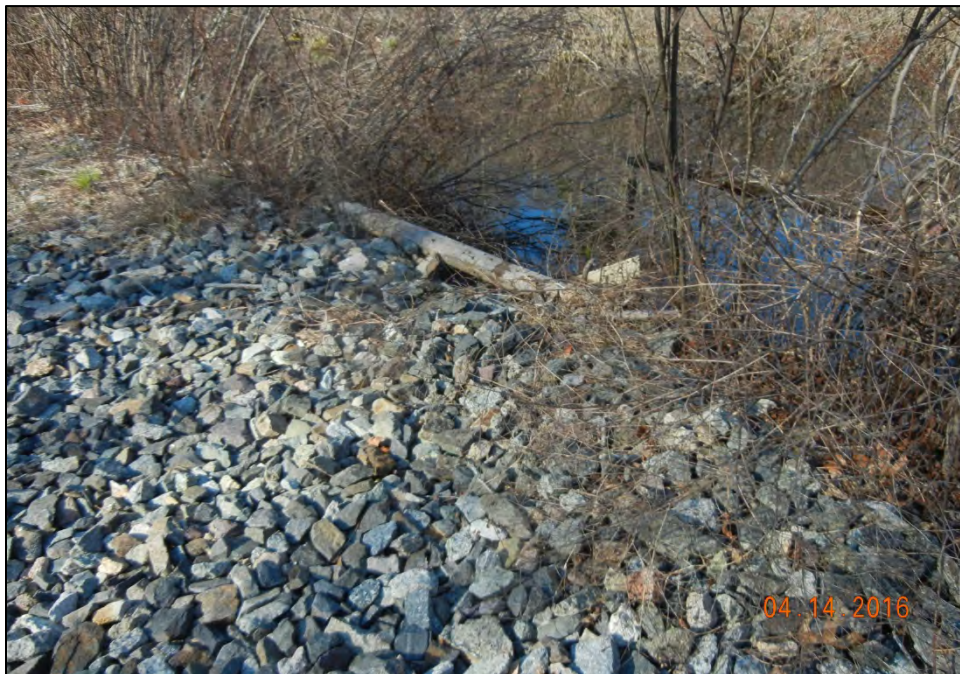
Photo No. 7 – Trap rock weir in railroad roadbed between northeast and northwest wetland (3,500 feet upstream of Kelsey Rd. culvert)
