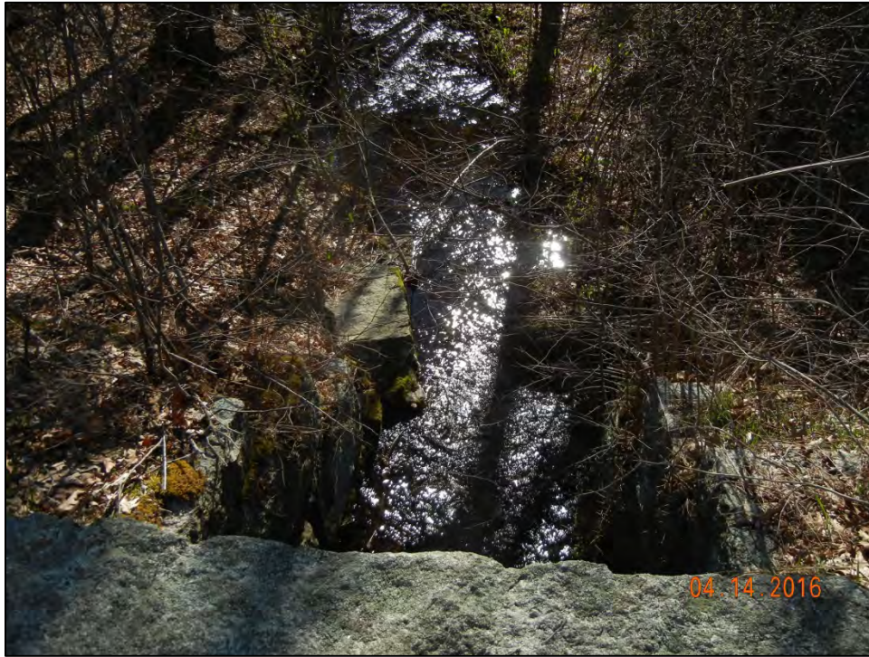
Photo No. 6 – Downstream railroad crossing (1,200 feet north of Lowe Pond)
