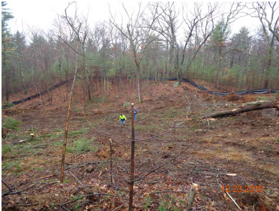
Photograph 2: Overview of the Enhancement Area while vegetation is being removed.
