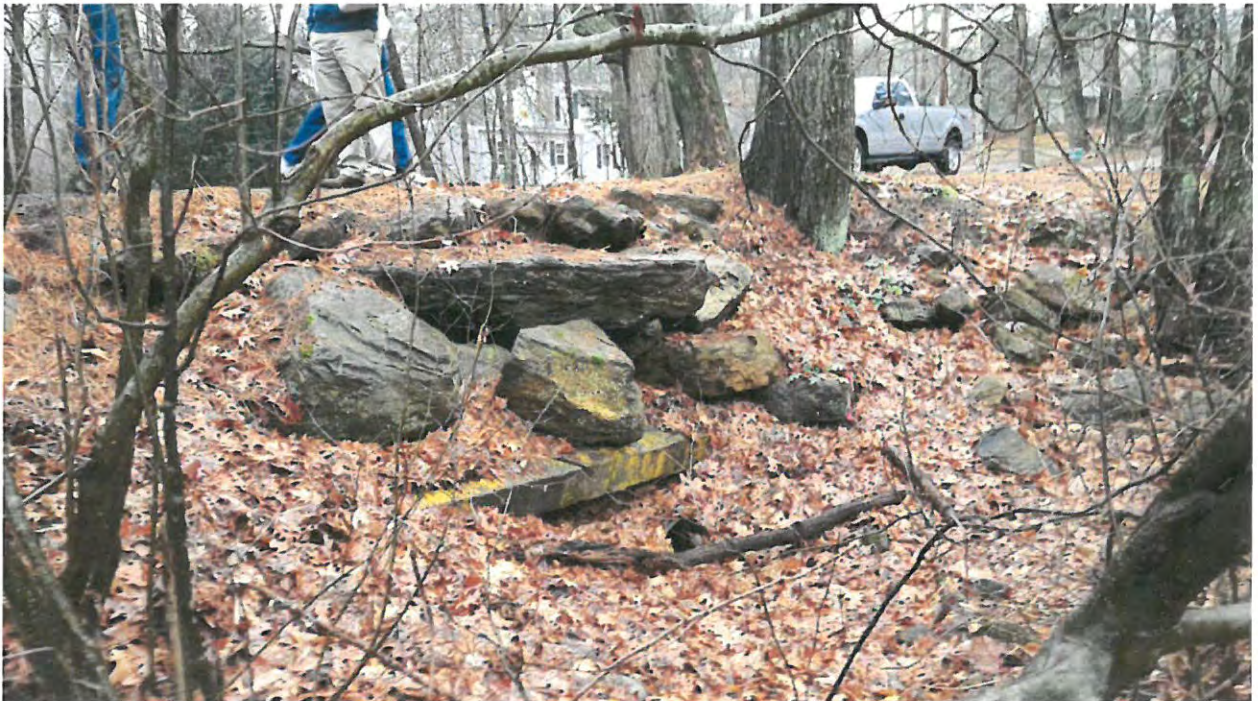
Photo B: Looking south towards upstream end of existing 12" CMP culvert
