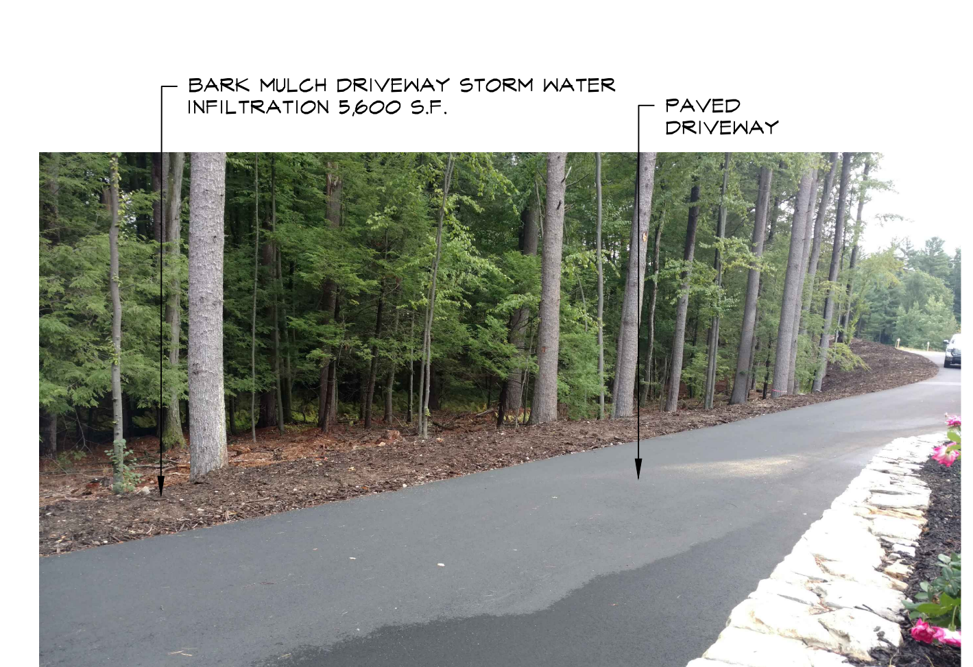
PHOTOGRAPH #8 DRIVEWAY AND BARK MULCH INFILTRATION
