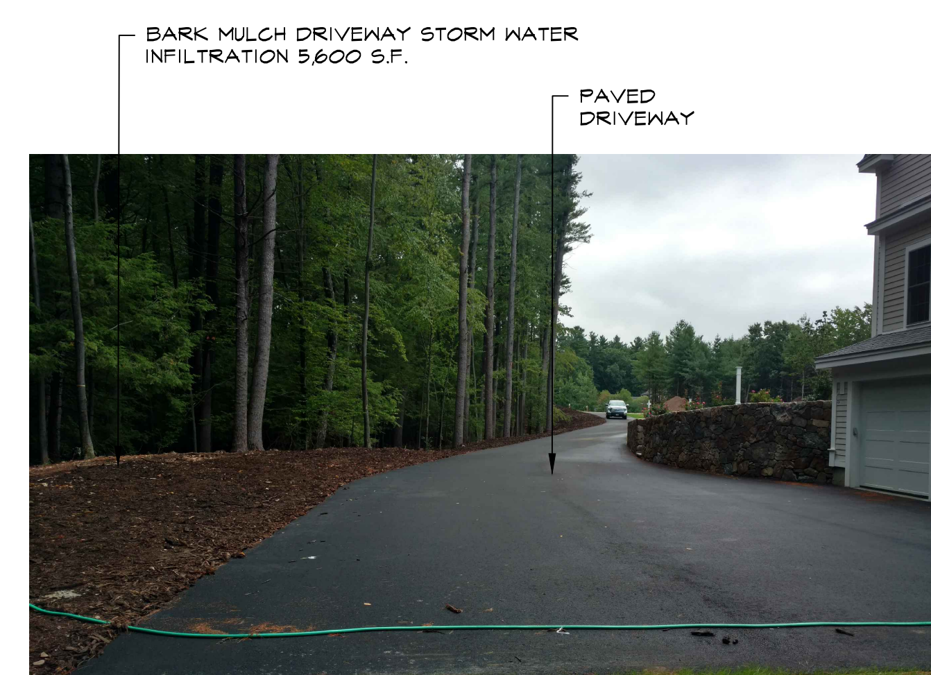
PHOTOGRAPH #7 DRIVEWAY AND BARK MULCH INFILTRATION
