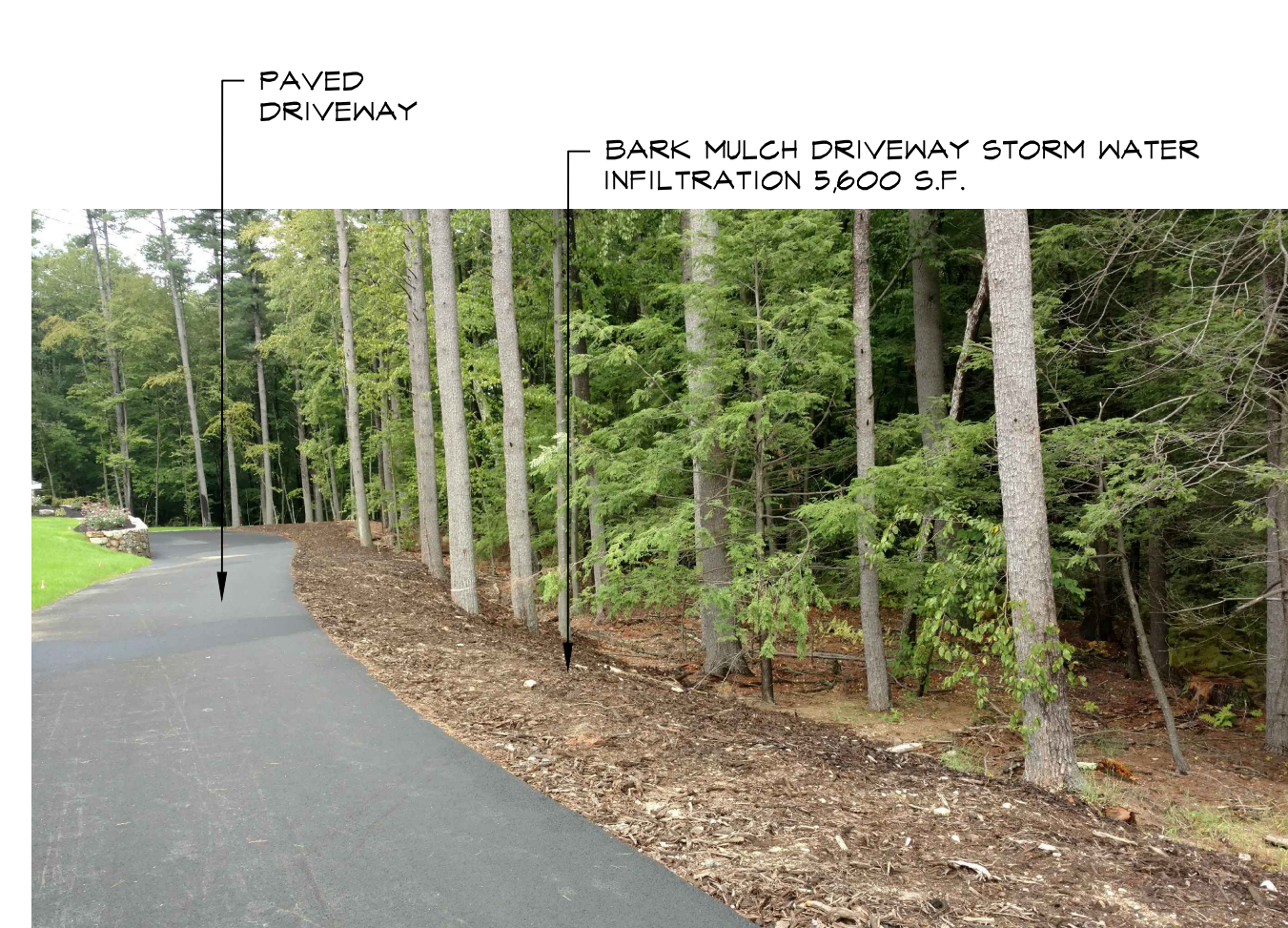
PHOTOGRAPH #2 DRIVEWAY AND BARK MULCH INFILTRATION
