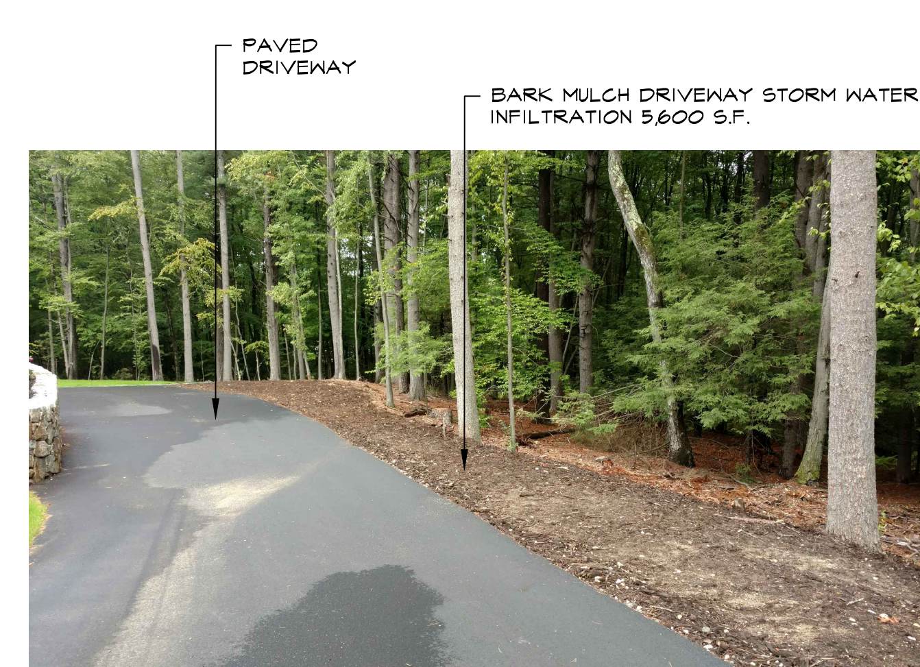
PHOTOGRAPH #3 DRIVEWAY AND BARK MULCH INFILTRATION
