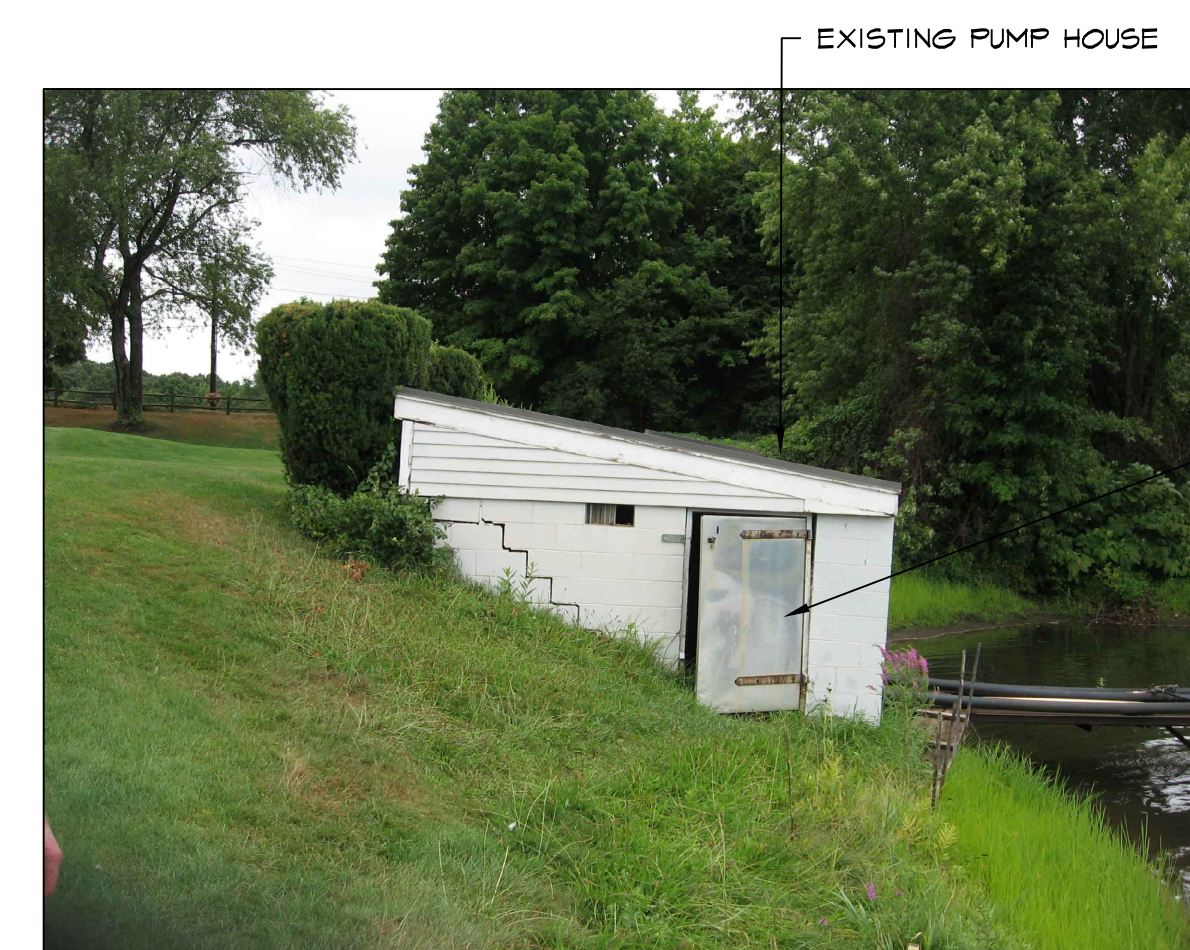
PHOTOGRAPH #4 EXISTING PUMP HOUSE
