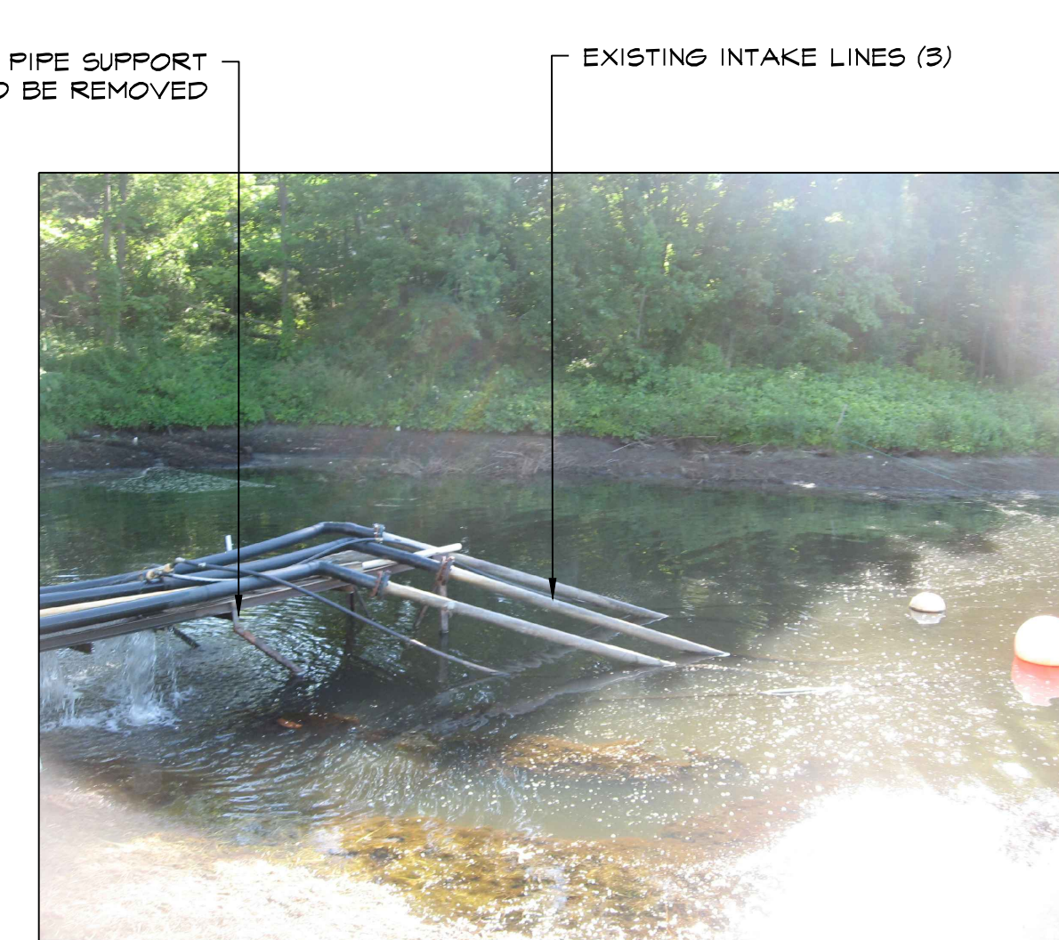
PHOTOGRAPH #8 EXISTING PUMP HOUSE INTAKES
