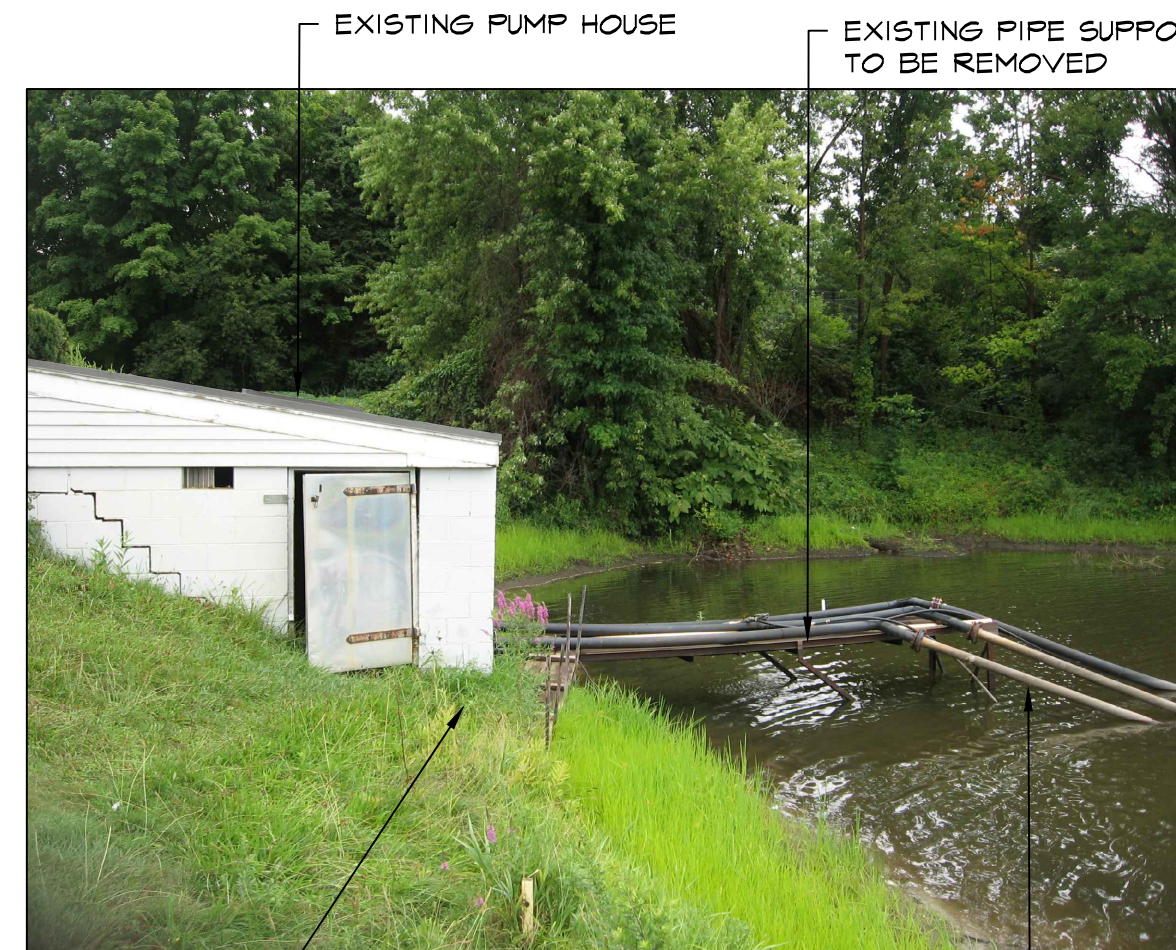
PHOTOGRAPH #2 EXISTING PUMP HOUSE & INTAKES
