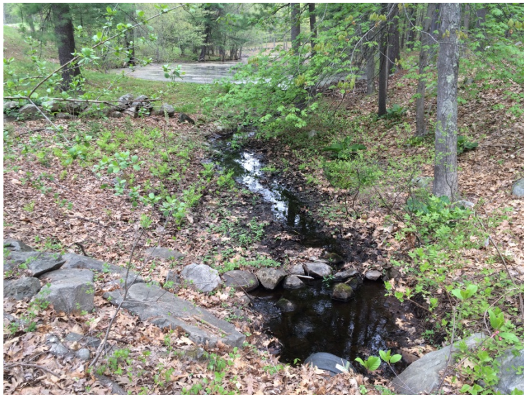
Photo 1: View upstream from driveway of dam and outlet channel
