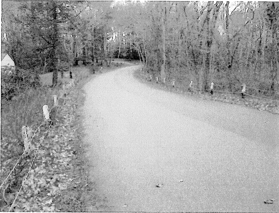
Photo A. Northerly view of Woodcrest Road where the existing culvert will be replaced. Photo by B. Prokop, November 25, 2014.
