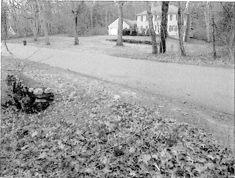
Photo A. Northerly view Woodcrest Road where the culvert is proposed for replacement. Photo by B. Prokop, December 3, 2014.
